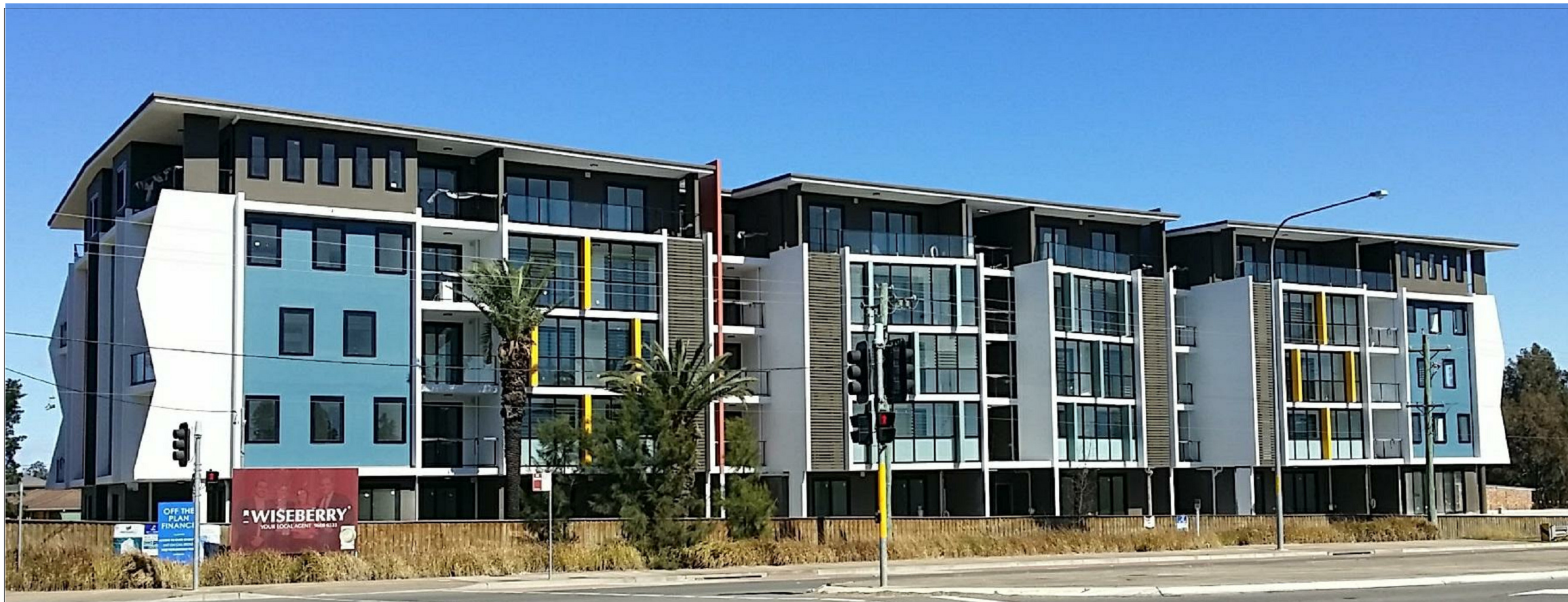
BUILDING A, LOT 5 - NEAR COMPLETION -
